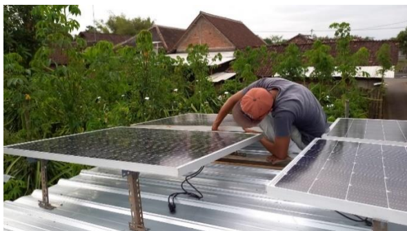
Gambar 2. Instalasi Panel Surya Gazebo 1
