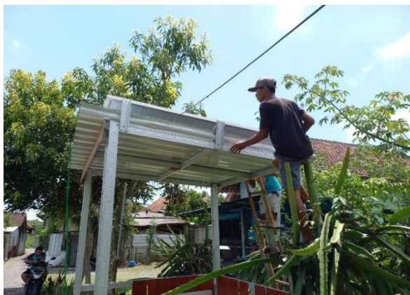
Gambar 3. Instalasi Panel Surya Gazebo 2
